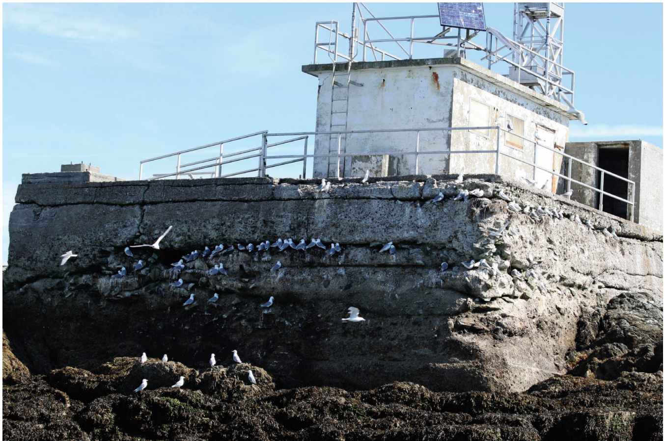
Fig. 2. Black-legged Kittiwake Rissa tridactyla nests at the Holland Rock colony in the summer of 2021. The majority of nests were located on the rock ledge between the bedrock and the concrete foundation of the weather station, on the southern and western faces of the structure.
